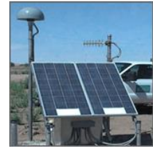
Solar array with GPS
